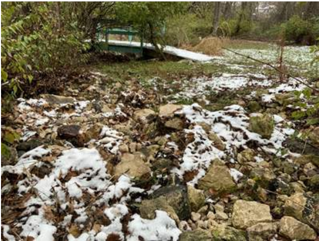
Typical drainage creek augmented with stone rip rap
