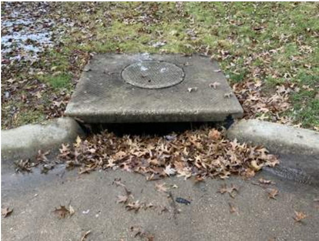
Typical catch basin in the concrete streets
