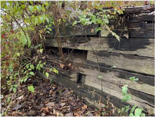
Deterioration in the retaining wall
