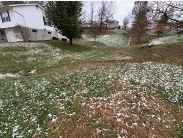
Typical drainage swale
