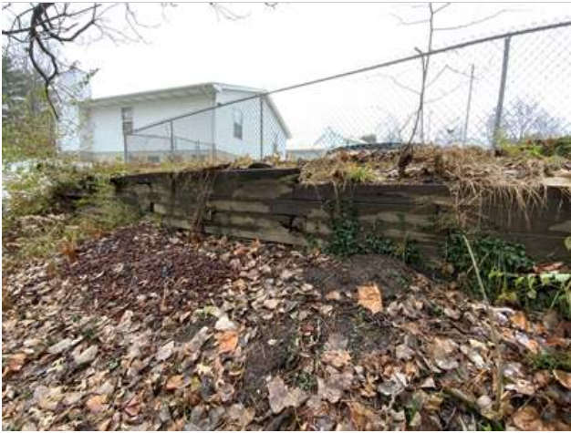
Wood tie retaining wall
