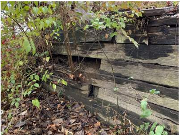
Deterioration in the retaining wall
